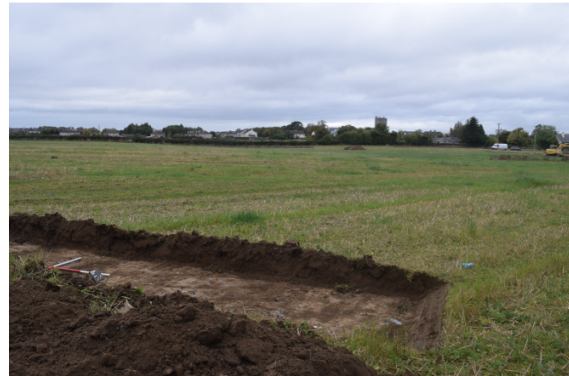
Plate 2: View of site from south-west corner. Looking north. Scales 1m & 1m
